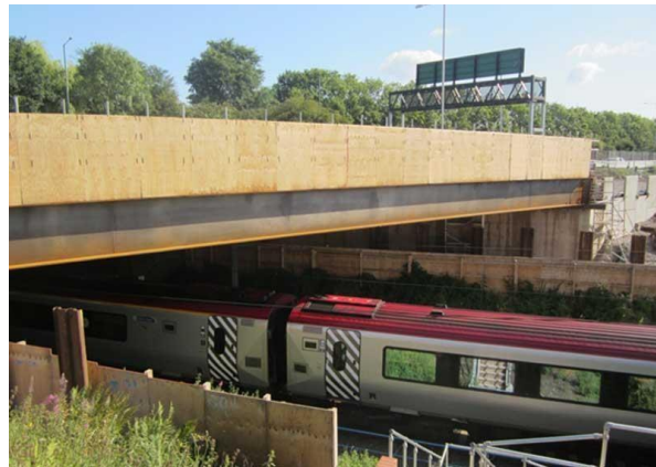
8.5 m for (rail road-bridge)
