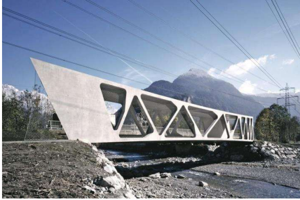
Figure 3.4-8: Concrete trusses with members under tensions.
